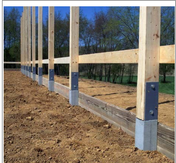
Illustration 5: Perma-Column Precast Piers
